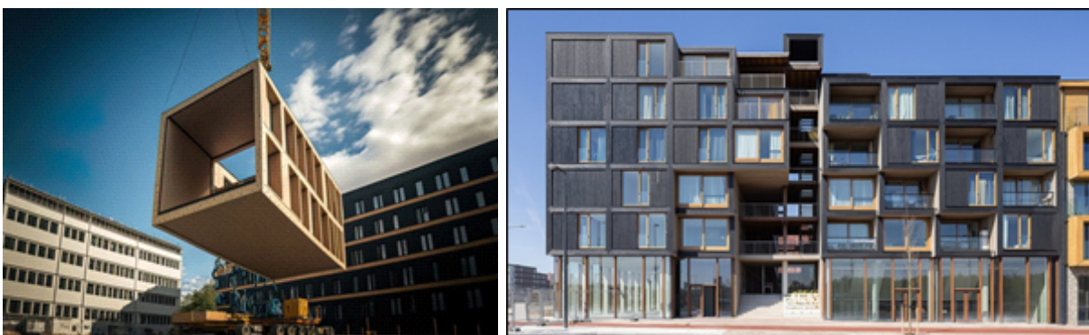
Figure 1 : Ongoing Construction of Modular Structure (left) and Constructed Modular Building (right)
