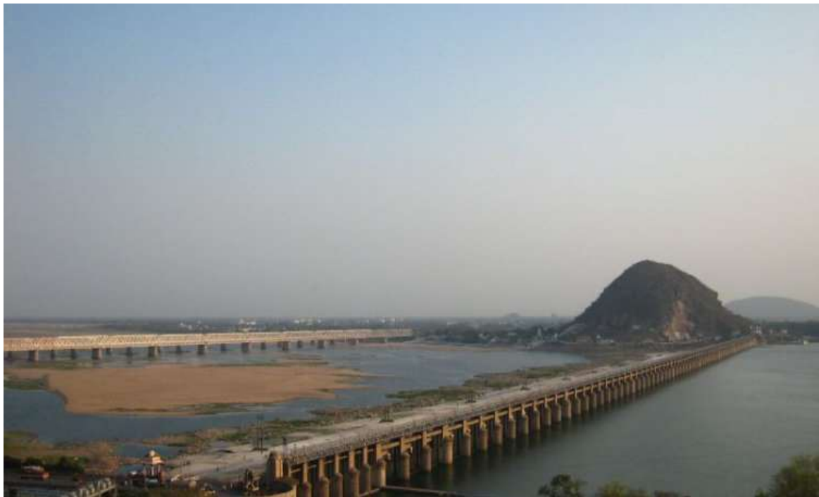
Fig : Vijayawada Dam
